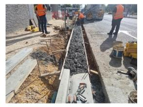
Works consist of improving the footpath by upgrading the asphalt with new flagstone pavers to match the existing street, replacing the existing damaged kerb and installing 3 new garden beds. The building owner will then plant and maintain their own plants.
