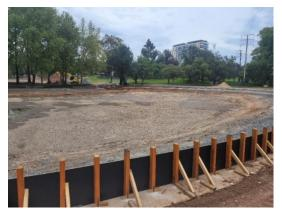
Bulk excavation within the lake is now complete, with final trimming of the lake subbase underway.
